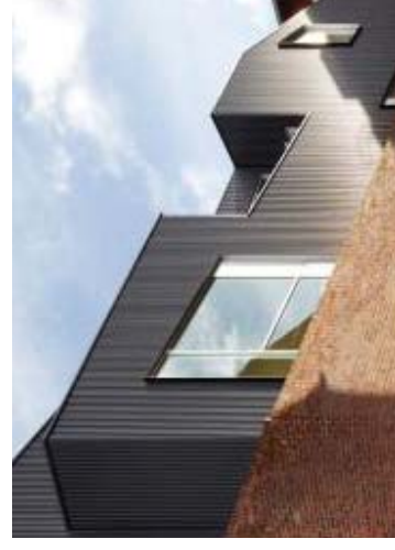
4 Powder coated aluminum profiled sheet cladding 192 Shareham Street, Sheffield UK (Project Orange)
